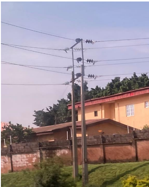
Figure 5-6.10 Raising poles by angle
