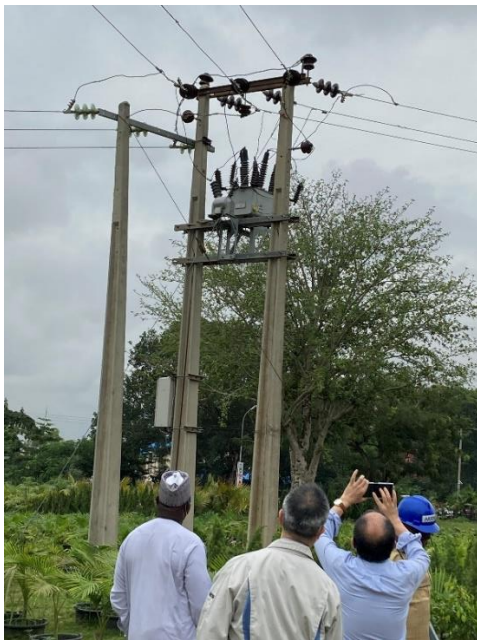
Figure 5-3.1 33kV recloser
