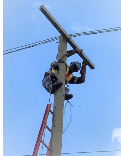
Figure 5-4.15 Replaced with FRP arm
