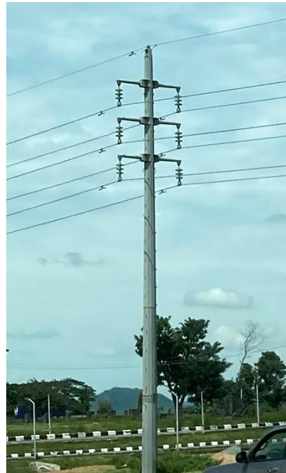
Figure 5-6.6 33kV line with transmission line specifications
