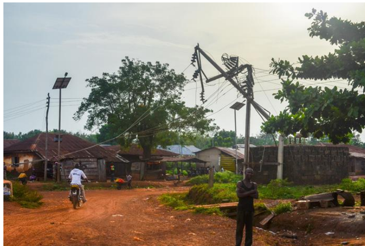
Figure 5-5.2 Broken pole due to insufficient strength
