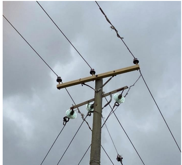
Figure 5-6.13 Repair of broken conductor on an 11kV line
