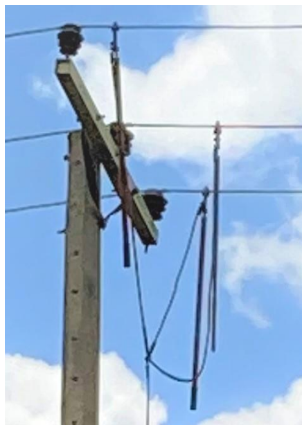
Figure 5-4.13 Installation of short-circuit grounding device
