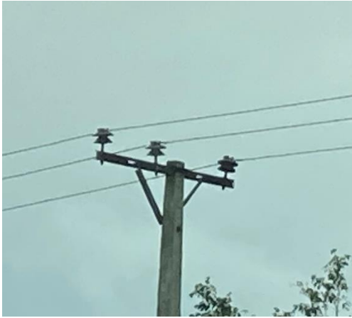
Figure 5-6.3 Standard arrangement for straight line
