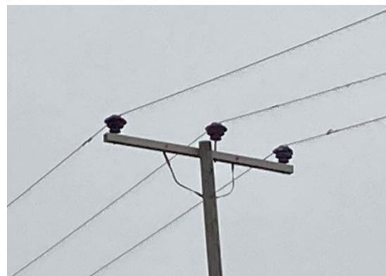
Figure 5-6.15 Substandard arrangement (Tie strap)
