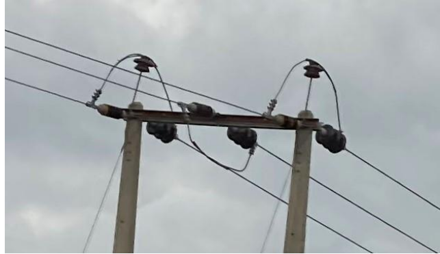
Figure 5-6.4 Jumper connection
