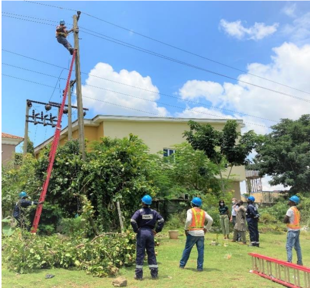
Figure 5-4.11 Fault facilities restoration site
