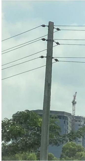
Figure 5-6.7 New type (arrangement) low-voltage pole
