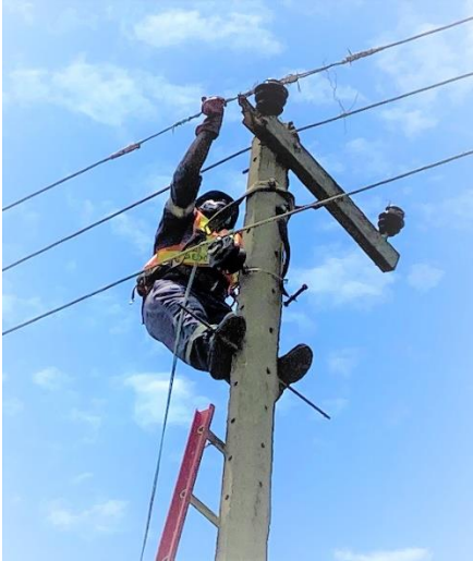
Figure 5-4.14 Removal of damaged arm
