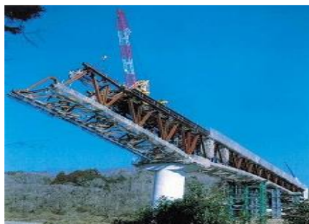
Figure 18.7-2 Traveler Crane Election PC-I Girder
