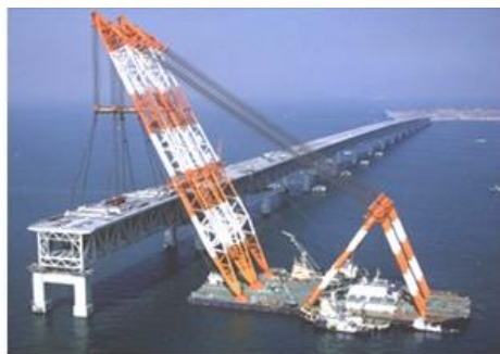
Figure 18.7-1 One Span Election using Jumbo Crane Steel Box Girder
