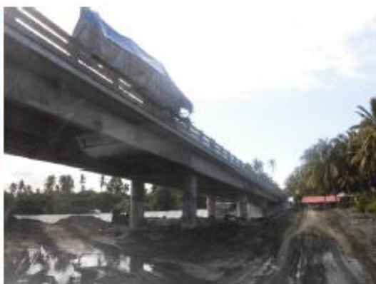
8. Masao Bridge under construction
