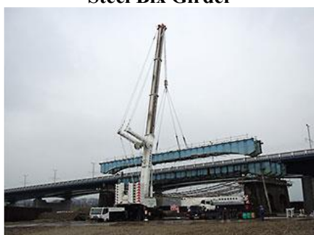
Figure 18.7-3 Track Crane Election for Steel Box Girder and PC-I Girder
