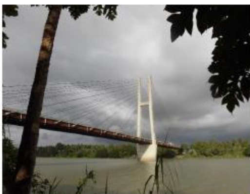
11. Agusan Bridge 2 (Cable-stayed Bridge)
