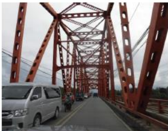
1. Old Truss Bridge over Agusan River
