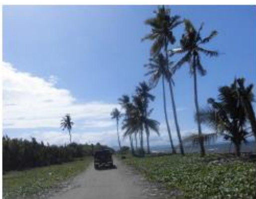
7. Existing Road along the coast
