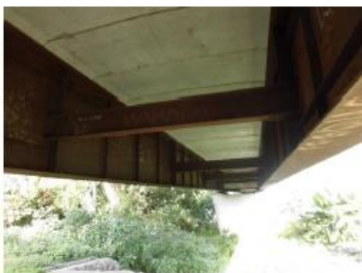
12. Approach Section of Agusan Bridge 2 (2-Main Girder Type of Bridge)
