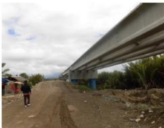
5. Banza Bridge 2 under construction
