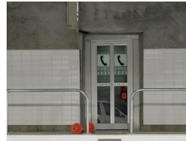
Emergency Telephone Box
