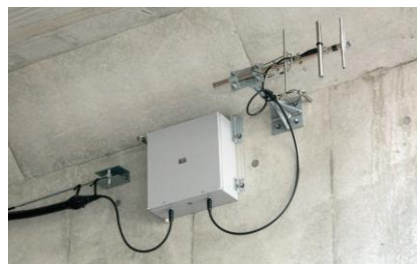
Photo 16.5-10 Wireless Radio System
