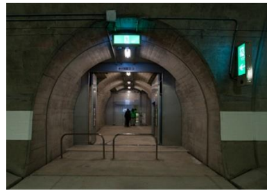
Evacuation Route (Evacuation Connection Tunnel)
