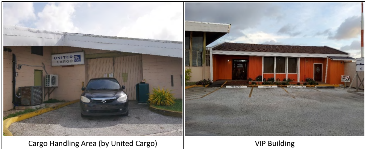
Figure 4-1-17 Current Conditions of United Cargo and VIP Building
