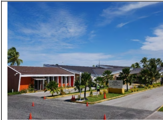
Exterior of Terminal Building (View from Airside)
