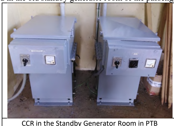
Figure 5-2-9 Existing Constant Current Regulators at VAV
