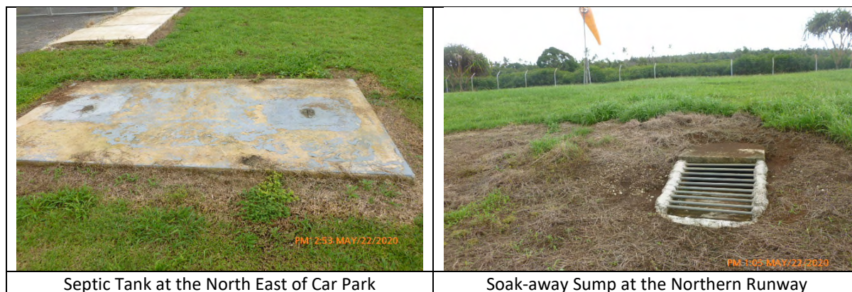
Figure 5-2-6 Sewerage and Drainage System at VAV
