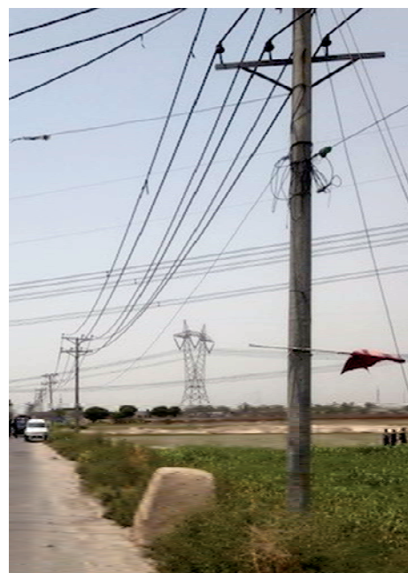
11kV distribution lines and poles
