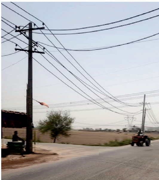
11kV distribution lines and poles
