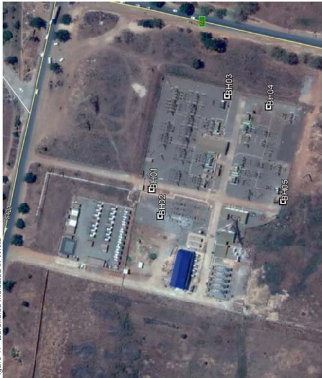
Figure 1: Boreholes Indicated in White
