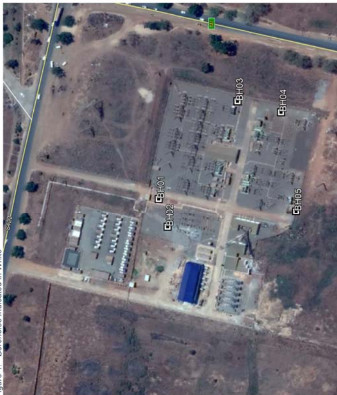
Figure 1: Boreholes Indicated in White
