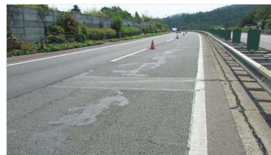
Cracks on Composite Pavement with weak base course
