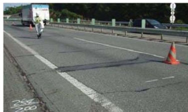
Cracks on Composite Pavement with weak base course
