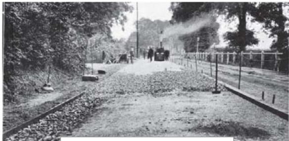
Asphalt Macadam 補修
