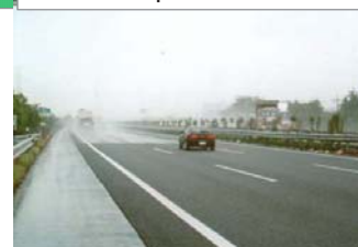
Porous Asphalt Pavement
