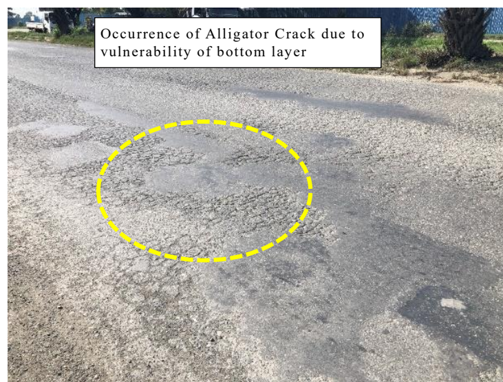
Figure 2.11 Alligator Cracks
