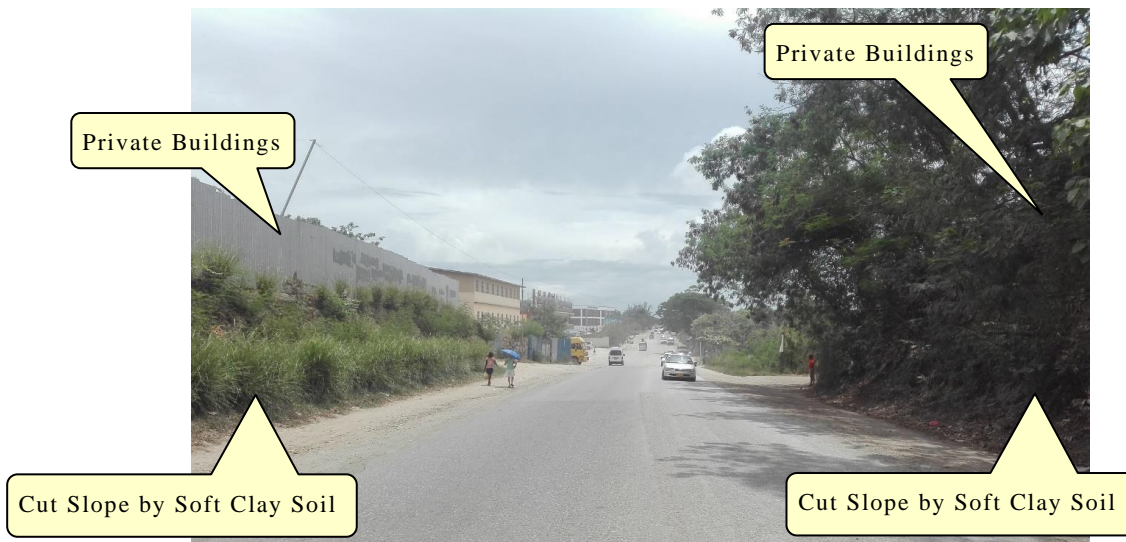
Figure 2.52 Cut Section from STA.4+540 to 4+680
