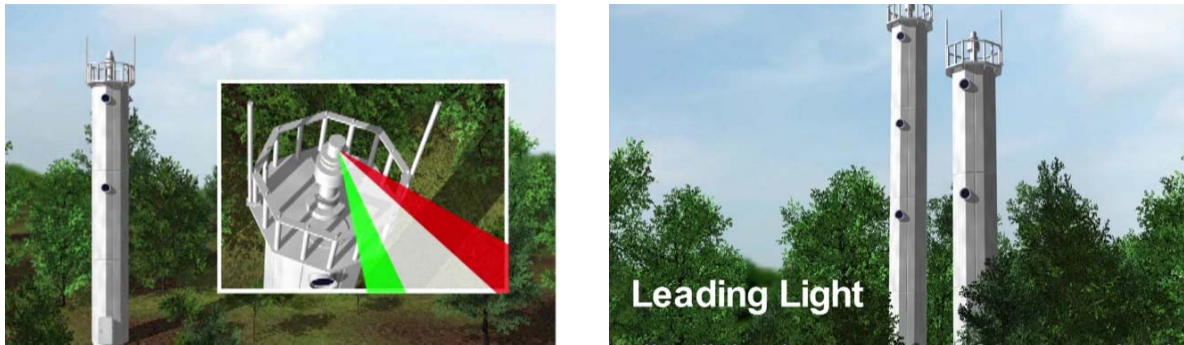
Figure 2-3 Image of the Light Tower
