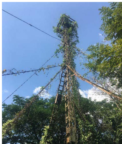
Photo: The Existing Thanlyin Point (Front) Light Tower
