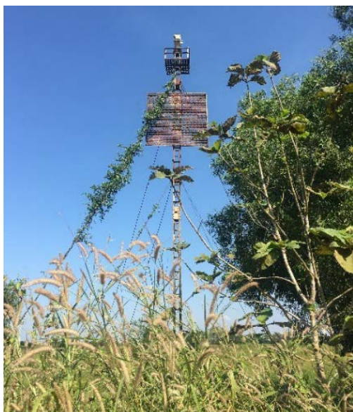
Photo: The Existing Thanlyin Point (Back) Light Tower
