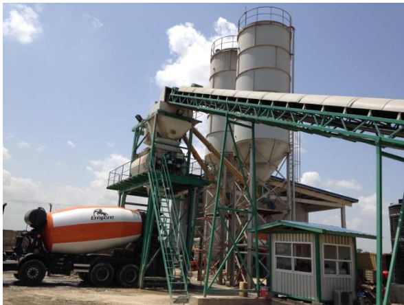
Photo 2.2-1 Concrete Plant in Production
