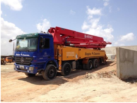
Concrete pump vehicle
