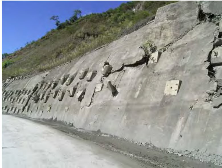
Photo.1.1 Failure example of mass movement countermeasure
