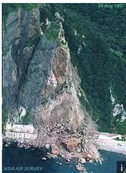
T3 Rock mass failure
