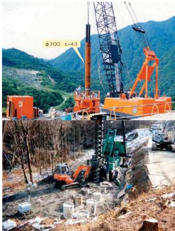
Photo. 4.2 Execution of pile work of steel pipe for mass movement prevention in Japan
