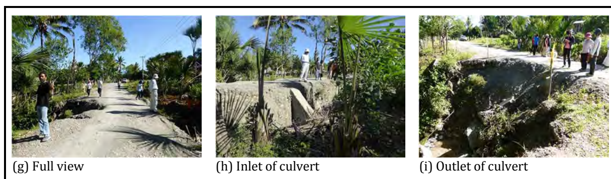
Figure C — Site conditions on 23/02/2017
