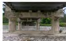
Figure 3. Mola bridge abutment 2011
