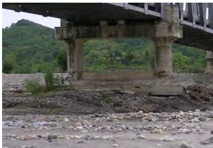
Figure 5 — Mora Bridge Pier 2011
