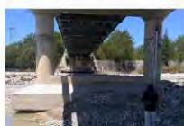
Figure 2. Sahen bridge pier 2017
