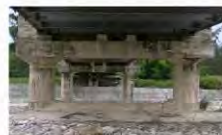
Figure 3. Mola bridge abutment 2011
