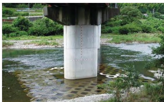
Figure 21 — Foot protection blocks in Japan
