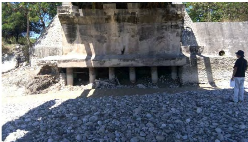
Figura 2 — Abutmen Ponte Sahen 2017
