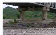
Figure 4. Mola bridge abutment 2011
