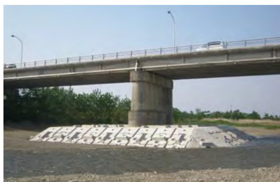
Figure 22 — Foot protection blocks in Japan
