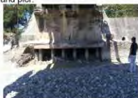
Figure 1. Sahen bridge abutment 2017
