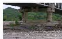
Figure 4. Mola bridge abutment 2011
