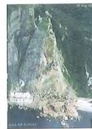
T3 Rock mass failure
