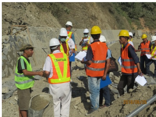
Safety patrol of masonry retaining wall on Ex-Japan Road (26 June, 2018)
