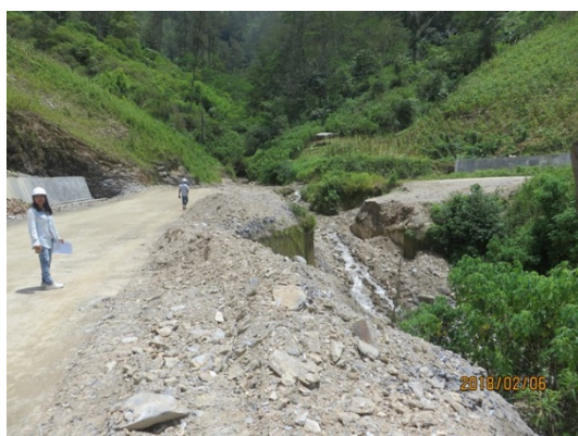
Condition of the proposed site for cross drainage on Ex-Japan Road
