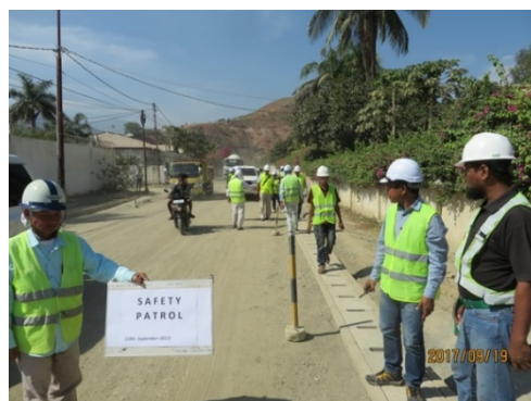
Safety patrol of the Construction of the Upriver Comoro Bridge (19 September, 2017)
