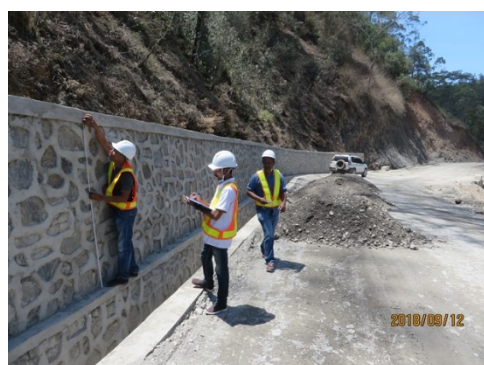
On-the-job training using checklists for masonry retaining walls on Humboe–Letefoho emergency repair work (12 September, 2018)
