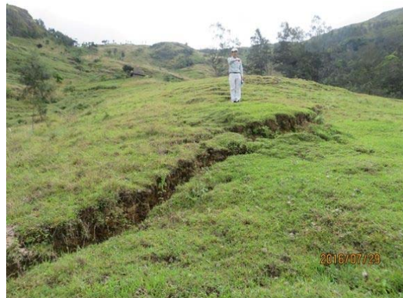
Scarp (long, steep slope) suspected of landslide
