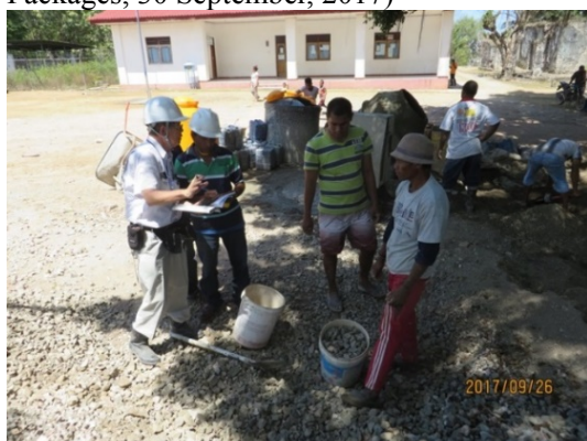
OJT for quality control of concrete mixes on Iliomar and Lospalos sites on the A08 road (No. 1 of 9 Packages, 26 September, 2017)
