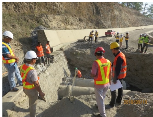
Safety patrol of laying of cross drainage on Ex-Japan Road (19 September, 2018)
