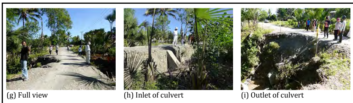
Figure C — Site conditions on 23/02/2017
