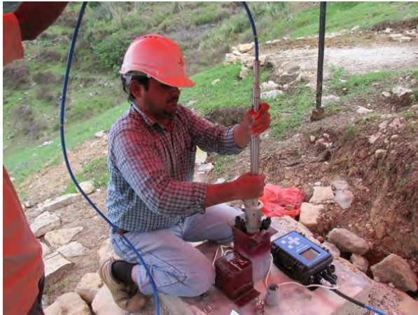
Figure 21 — Insertion of the probe of the inclinometer into the casings
