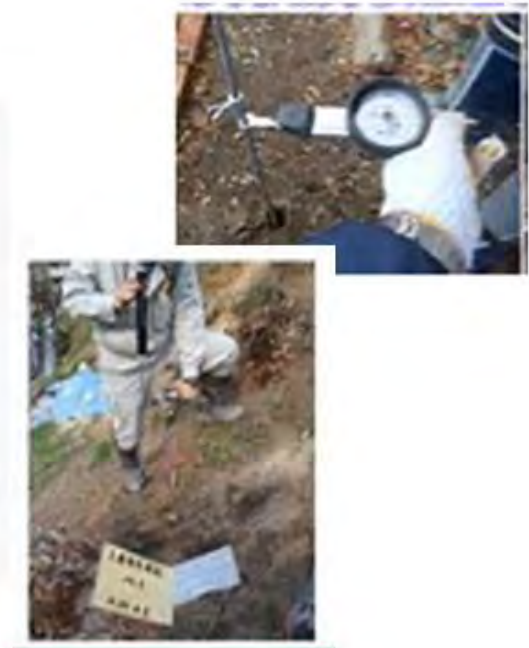
Figure 4.4 Penetration tests by man power
