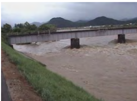
Figure 9 — Hydraulic phenomenon around bridge piers (Japan example)
