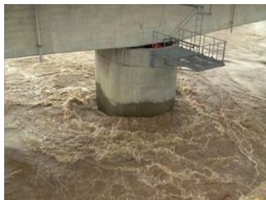
Figure 9 — Hydraulic phenomenon around bridge piers (Japan example)
