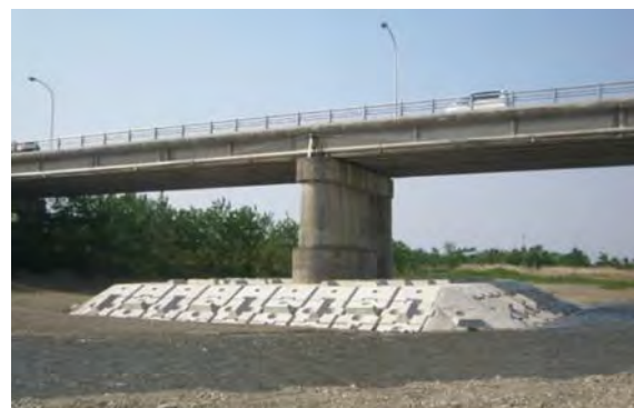
Figure 22 — Foot protection blocks in Japan
