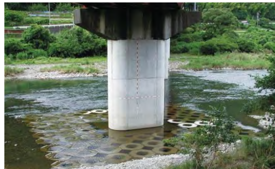
Figure 21 — Foot protection blocks in Japan
