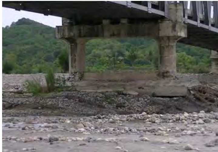
Figure 5 — Mora Bridge Pier 2011
