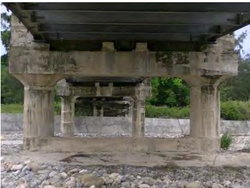
Figure 4 — Mora Bridge pier 2011
