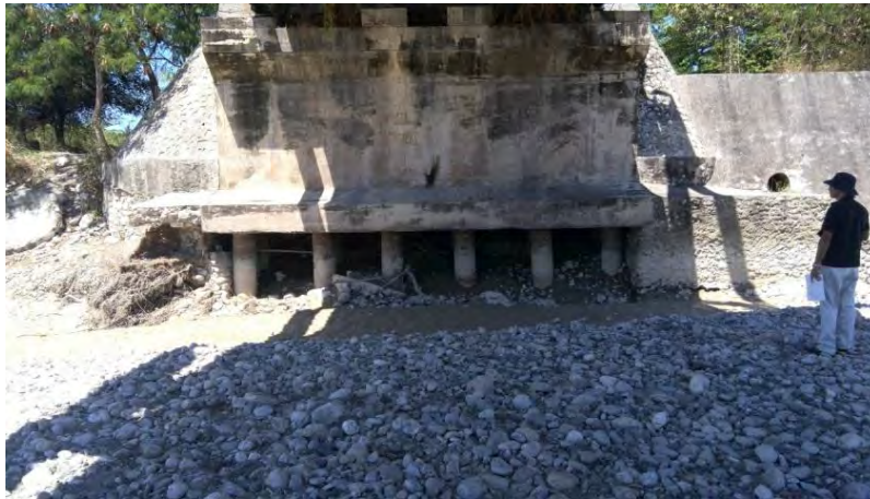
Figura 2 — Abutmen Ponte Sahen 2017
