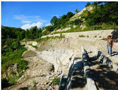
Embankment slope failure on A07 due to the unsuitable foundation material and lack of compaction
