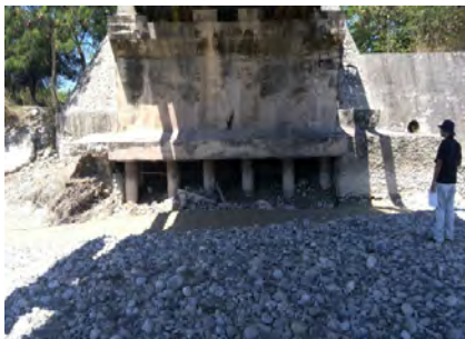
Scouring of bridge substructure on A14 due to severe river flow and lack of protection
