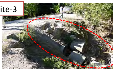
Site-3: Damaged Culvert in Sesurai
