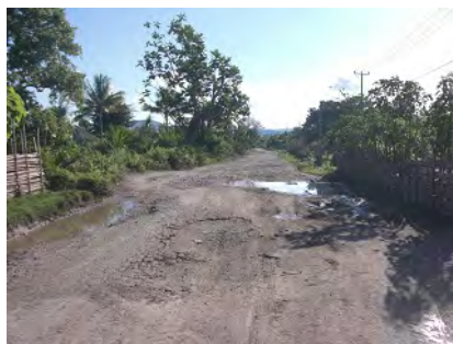
Pavement collapse on A05 due to the lack of roadside ditch
