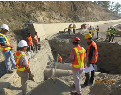
Ph-4: Ditto but Inspection site ②: STA 6+270 , RC double Pipe Culvert, half of the road open to Public Traffic
