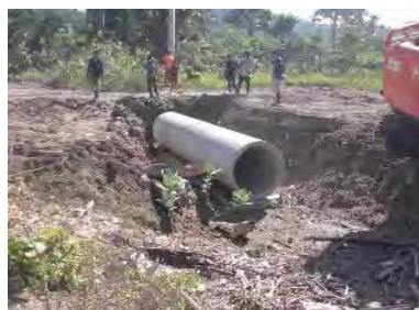
No.4_9 Packages, Betano Pipe Culvert installation, Foundation ground condition must be checked @2017.08.16
