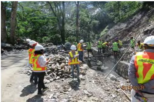
Ph1: STA0+300 A10 from Humboe JCT, Stone Masonry Retaining Wall is constructing.
