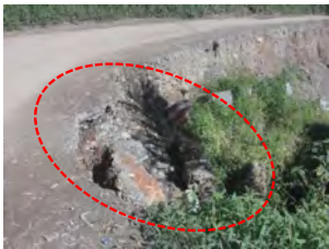
Damaged Shoulder
