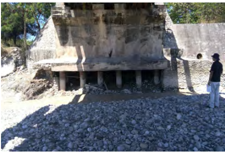
Scouring of bridge substructure on A14 due to severe river flow and lack of protection
