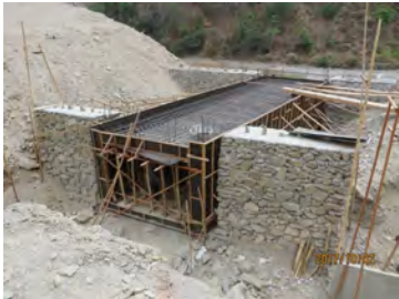
Box Culvert at STA 12Km+065 on Ex-Japan Rd.: 2.0*2.5m, both side with Sone Masonry Wall, L=12m @2017.10.02
