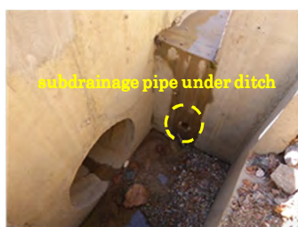
Subdrainage pipe under roadside ditch
