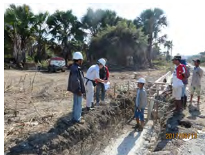
Stone Masonry Line Drain: Due to a little gradient 0.35%(upper stream) and 0.25% (near out-let), instruction was made for most attention setting the elevation line @2017.09.30
