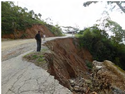
Cut & embankment slope failure on A02 due to the heavy rain and lack of slope protection
