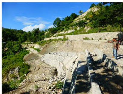
Collapse of embankment slope on A07 due to the unsuitable foundation material and lack of compaction
