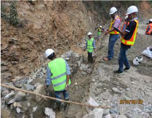
At STA 13km near existing Bridge, Stone Masonry Retaining Wall OJT held on 28 June 2018
