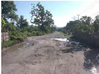
Pavement failure on A05 due to the lack of roadside ditch
