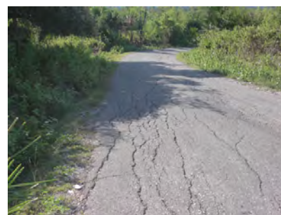
Alligator cracks on A05 due to the unsuitable base and roadbed material
