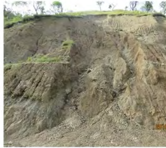
Surface layer collapse
