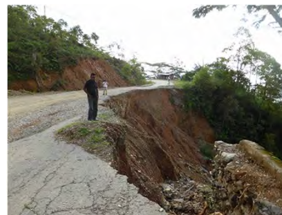
Collapse of cut slope on A02 due to the heavy rain and lack of slope protection
