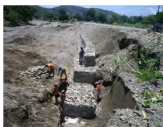
Rehabilitation of damaged revetment
