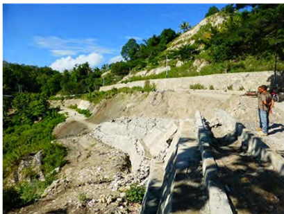
Embankment slope failure on A07 due to the unsuitable foundation material and lack of compaction
