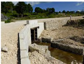
Scouring measure of cross culvert
