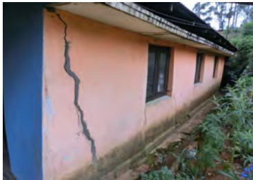
The house crack and deformation
