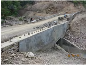
Ditto but Completed Box Culvert 2.5m*2.0m, as a Variation Order @2017.11.17
