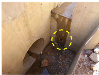
Sub-drainage pipe under a side ditch
