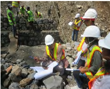
Ph2: Ditto but using, CL(Checklist)_SM Retaining Wall sheets. Inspecting according to each “check item” of the sheet.
