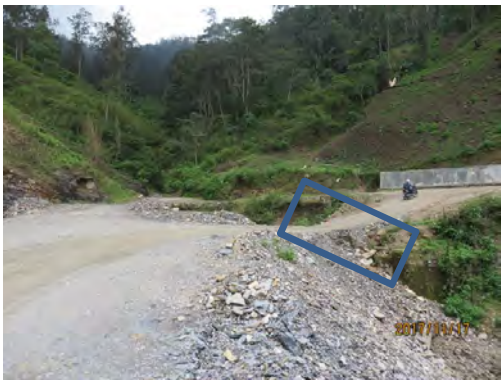
Box Culvert at STA 12Km+065 on Ex-Japan Rd.: 2.0*2.5m, both side with Sone Masonry Wall, L=12m @2017.10.02
