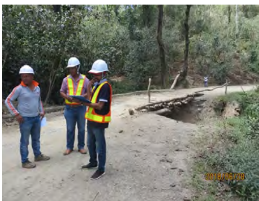
STA 18km (near Letefoho); Existing bridge had been destroyed by Flash Flood. RC pipe on site were inspected on OJT held on 28 June 2018
