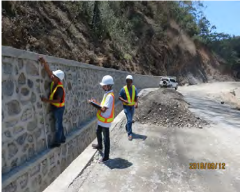
STA 13km, Stone Masonry Retaining Wall are inspected for completed part OJT using the Check List held on 12 September 2018
