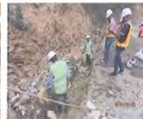
STA at about 13km near existing Bridge, Stone Masonry Retaining Wall. Checking Quality of the works using Check List for Construction: "Stone Masonry Retaining Wall" on 28 June, 2018 «Quoted from Ph5, memo No.19»
