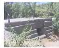
Gabion Box Retaining Wall. Existing steel corrugated pipe (2m dia) are used for remedial work. Some of old steel pile is found deformed from round shape on 13 February, 2018 «Quoted from Ph5, memo No.17»
