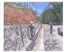
On-going construction area for Stone masonry Retaining Wall and Live Drainage on 13 February, 2018 «Quoted from Ph30, memo No.17»
