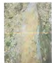
Figure 8.4 Erosion and weathering on the cut slope
