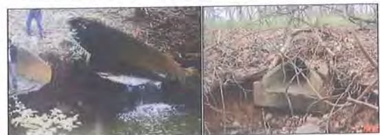
Figure 9.1 — Examples of erosion at culvert outlets (7)
