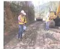
STA2-3 km Sub-Grade leveling and preparation for Sub-Base course; gravel material from Gileso River. And inspection of leveling and compaction by Macadam Roller on 28 June, 2018 «Quoted from Ph3, memo No.19»
