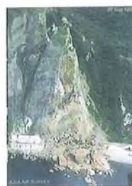
T3 Rock mass failure
