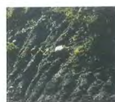
Figure 8.4 Erosion and weathering on the cut slope
