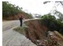
Cut slope failure on A02 due to the heavy rain and lack of slope protection
