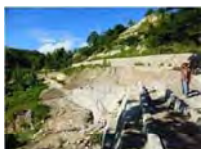
Landsliding slope failure on A07 due to the unsuitable foundation material and lack of compaction
