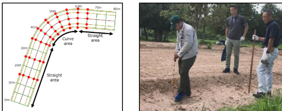
Fig. 48 Left: Position of Reference Pile, Right: Stakeout of Horizontal Position
