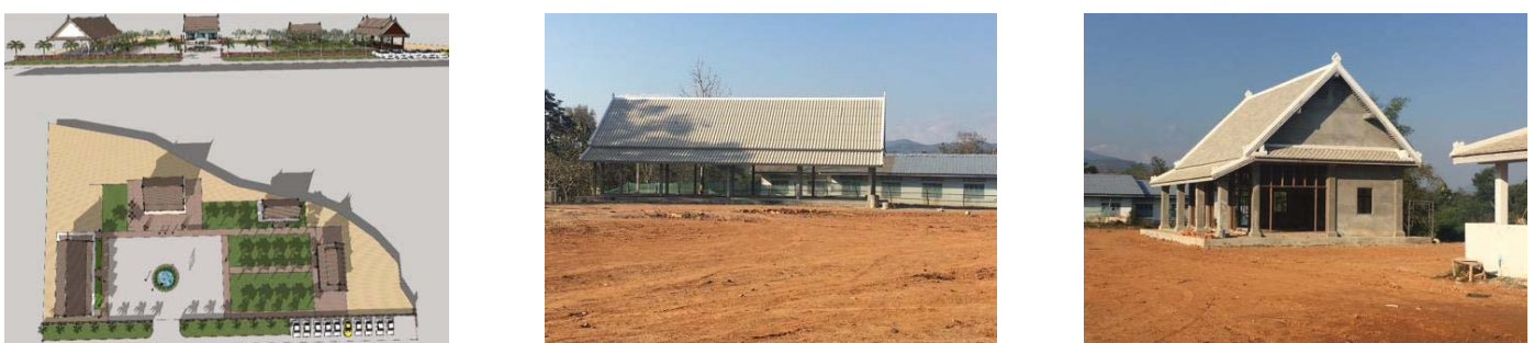
Pottery support facility under construction by ADB support (Pottery production experience program facilities are not included)
