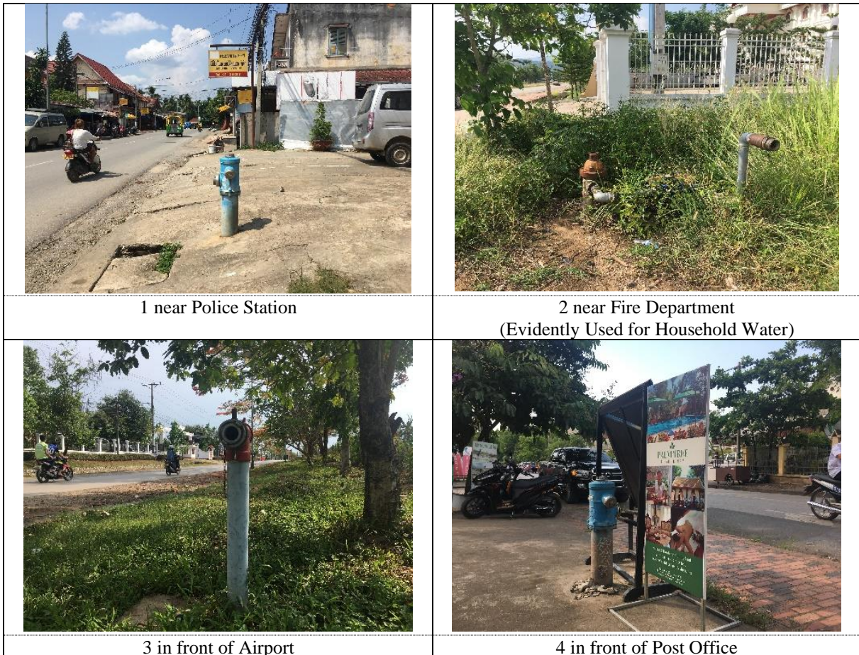
Figure 3.32: Status of Fire Hydrant Installation
