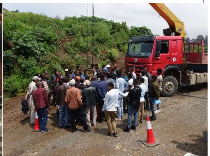
Photo 12 : Safety on Crane Works③
