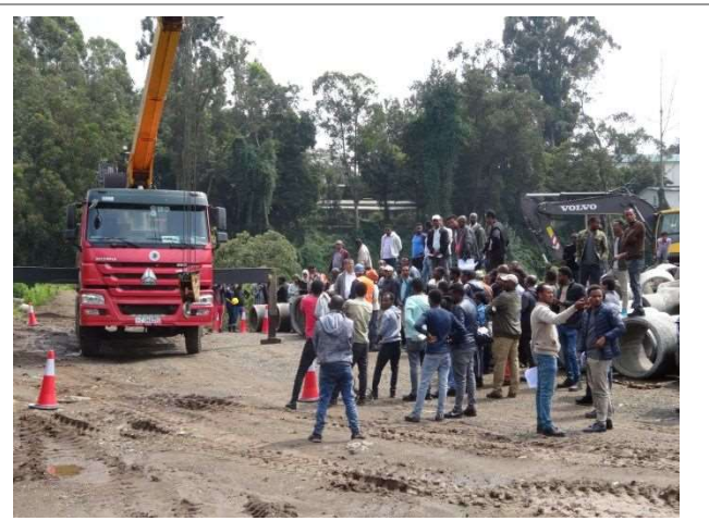
Photo 10 : Safety on Crane Works①
