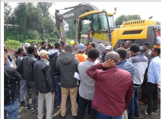
Photo 9 : Safety on Excavator Works②
