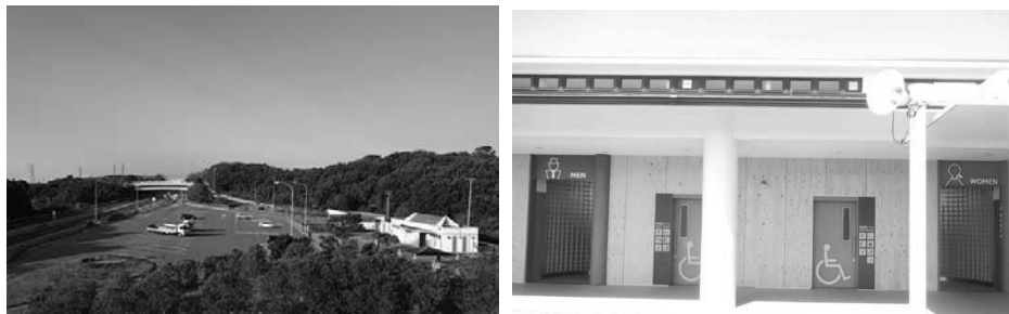
Source: Aichi Road Concession Co.,Ltd. HP
