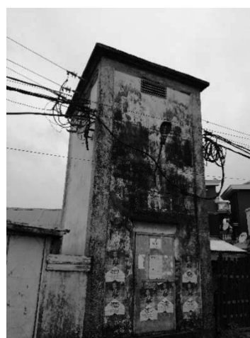
Figure 21.3.10 20kV/380V Substation
