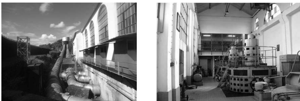
Figure 21.3.3 Volobe Hydropower Station
