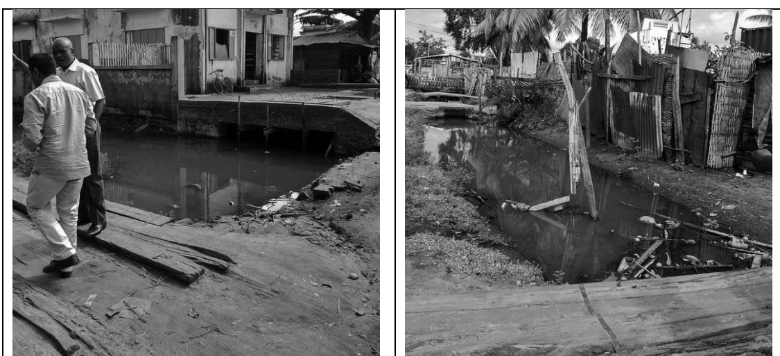
Photo 1 Under-dimensioned canals
