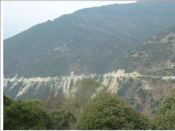
Photo 1: Slope failure along the Primary Highway (EW-1) in Tongsa
