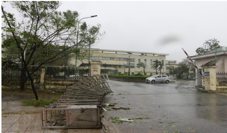
Photo 1. The district hospital is no longer operational after the typhoon
