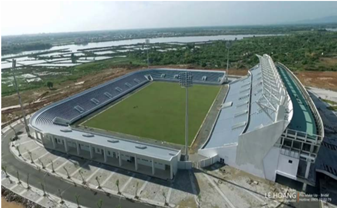
Photo 3. Panorama of Hoa Xuan stadium
