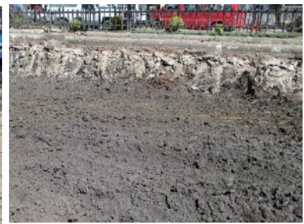
Excavation for Subgrade
