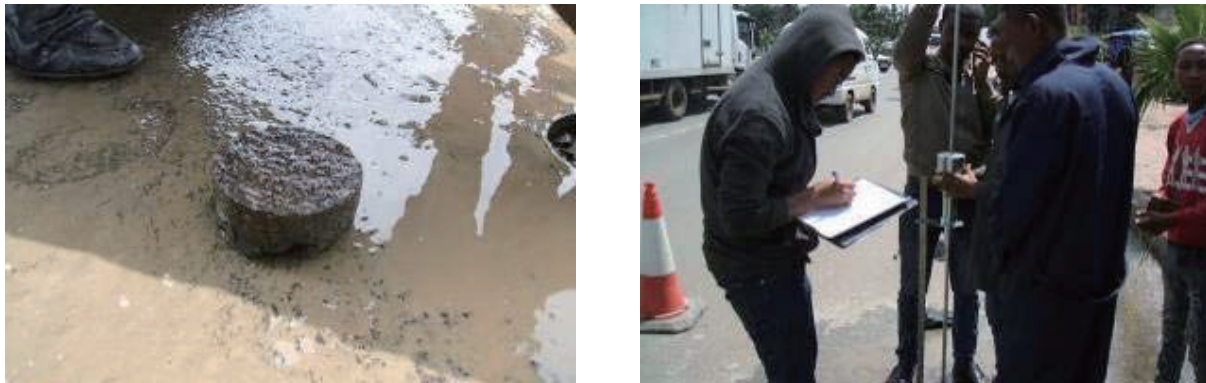
Figure 9 Photos on DCP Testing on Site (August 2017)
