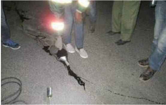
Crack sealing
