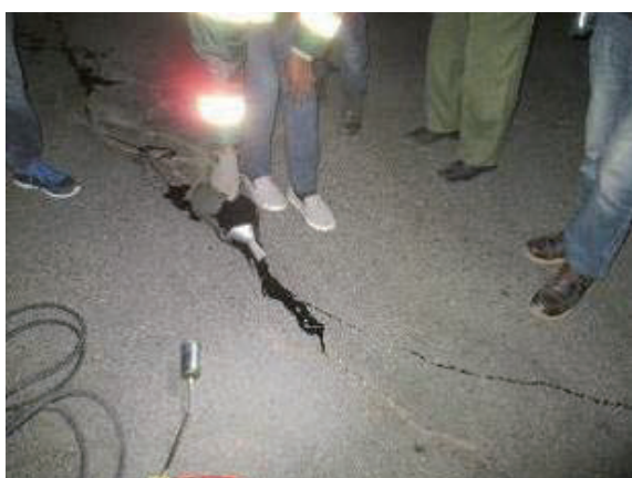
Crack sealing
