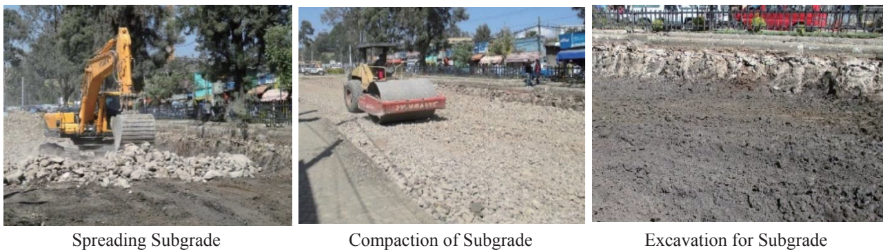
Figure 21 Photos of 2 nd Pilot Project
