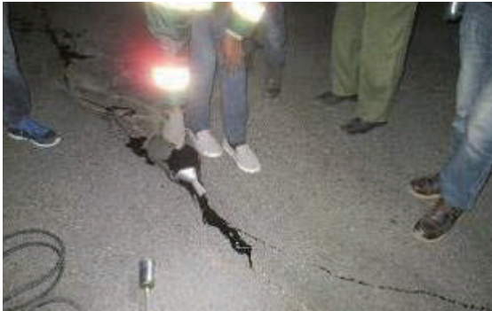
Crack sealing
