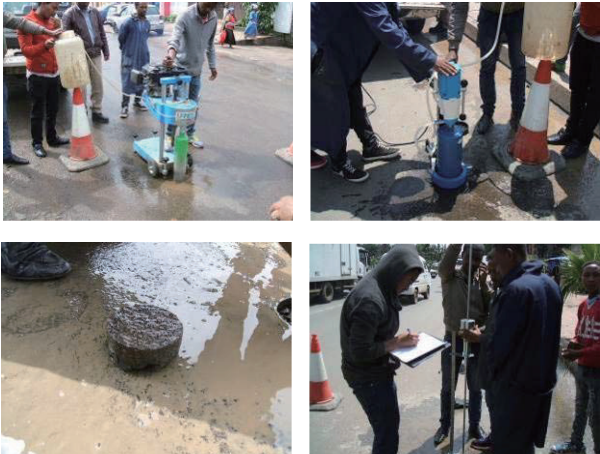
Figure 8 Photos on DCP testing on site (August 2017)
