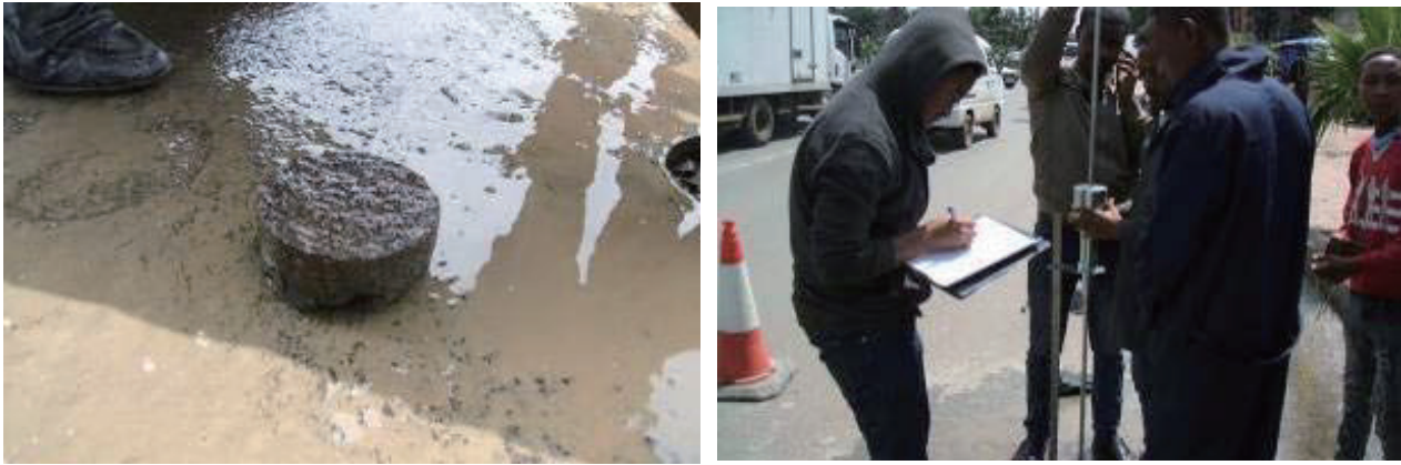
Figure 9 Photos on DCP Testing on Site (August 2017)
