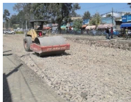
Compaction of Subgrade
