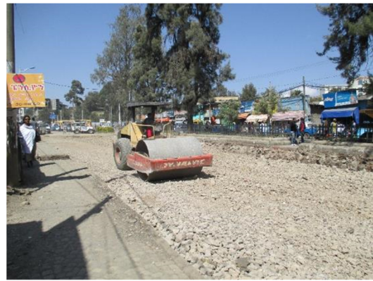
Compaction of Sub Grade
