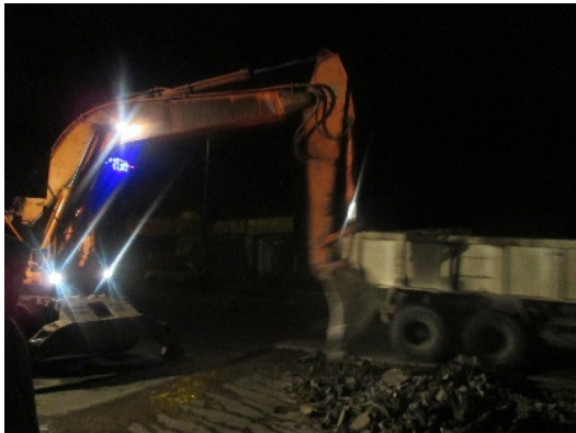
Asphalt Pavement Removal
