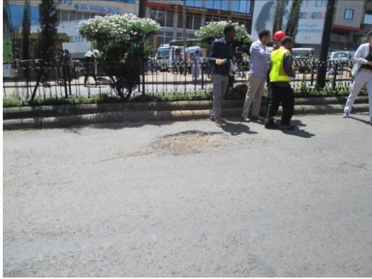
Before maintenance Work
