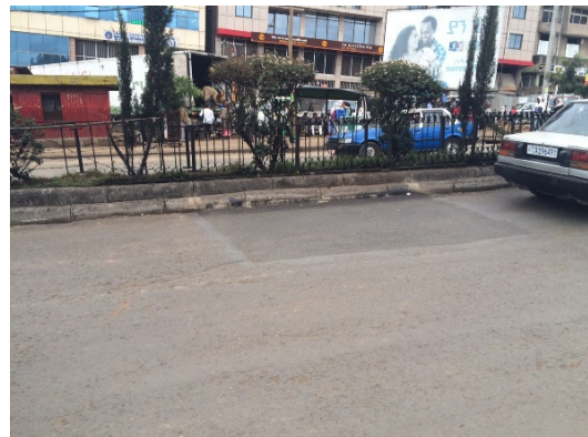
After Maintenance Work
