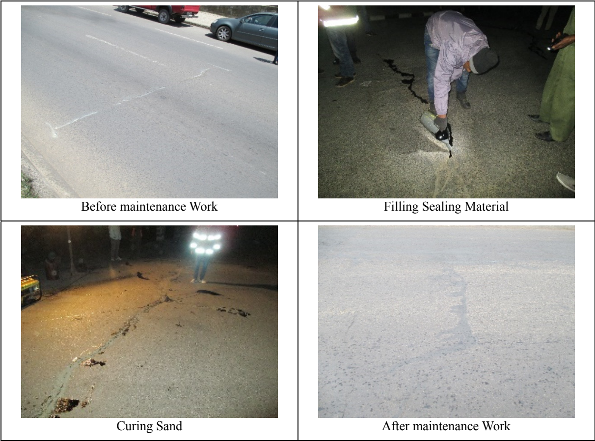
Figure 2-3-27 Photos of First Pilot Project (Crack Sealing)
