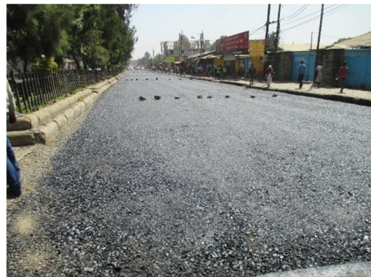
Establishment of Base Course
