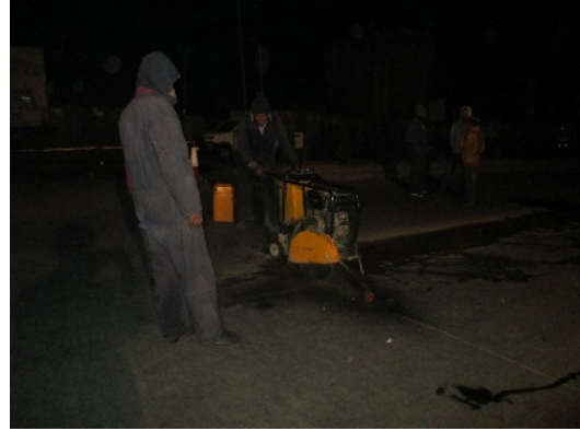
Asphalt Pavement Cutting
