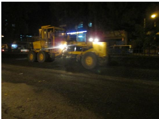
Establishment of Sub Base
