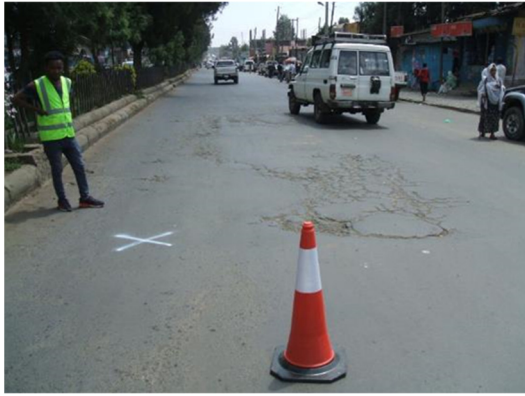
Before Maintenance Work
