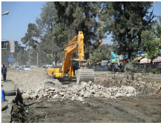
Establishment of Sub Grade
