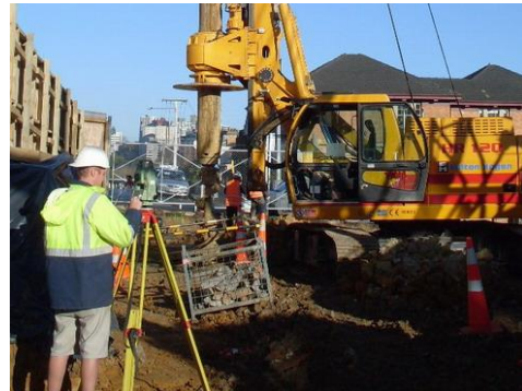
Figure 5.3-24 Survey for Drill
