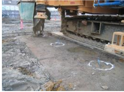
Figure 7.1-11 Pile Center Position
