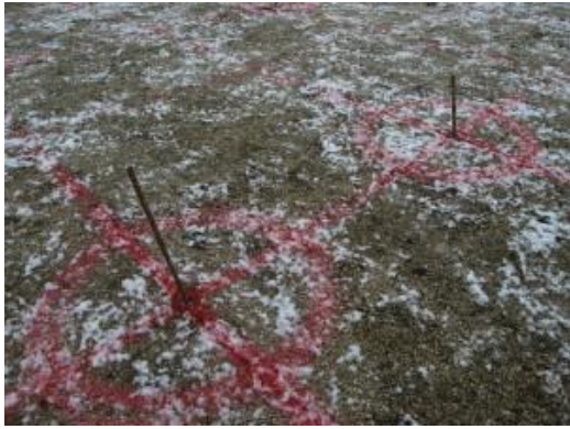
Figure 7.1-11 Pile Center Position
