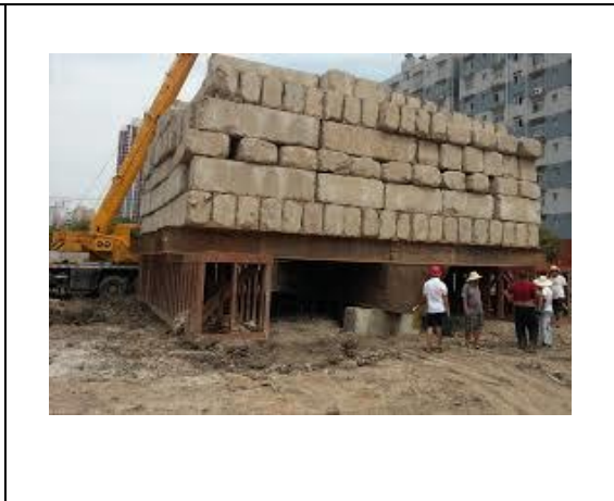
Figure 5.3-14 Static Load Test
