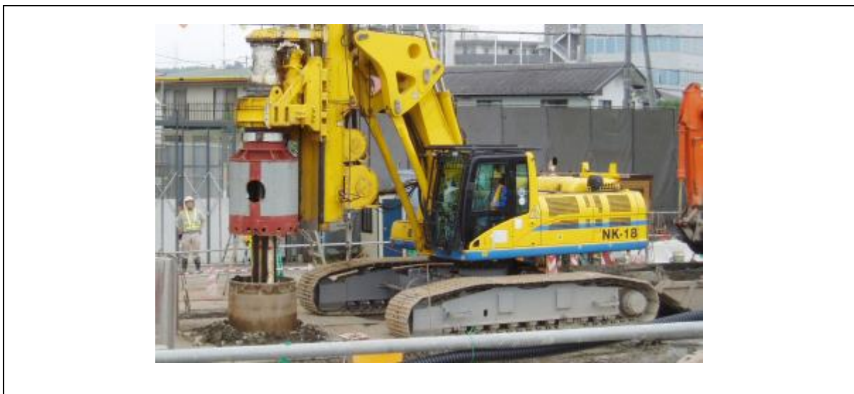
Figure 6.2-3 Excavation Machine for Earth Drilling Method
