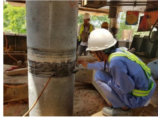
Figure 7.3-18 Welding Work Condition
