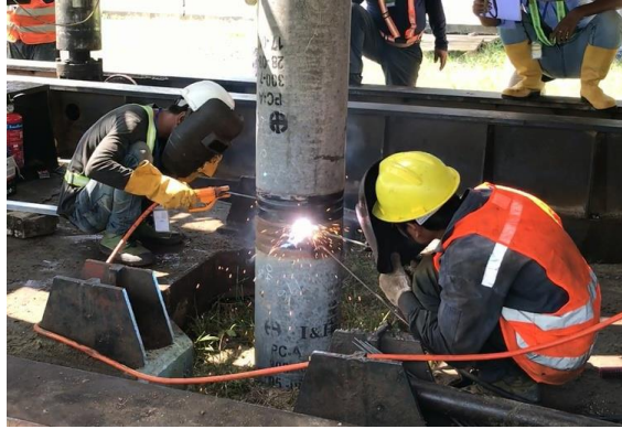
Figure 7.3-17 Welding Work Condition
