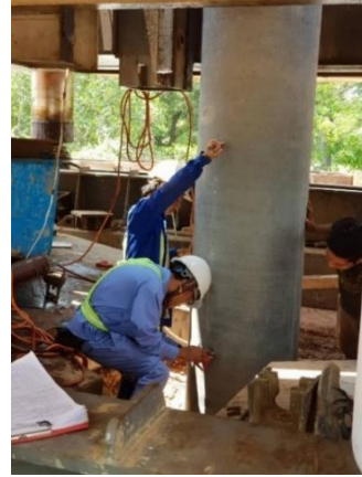
Figure 7.3-24 Measuring for Inclination
