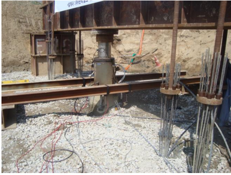
Figure 5.3-1 View of Static Loading Test
