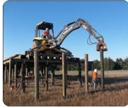
Figure 1.2-3 Timber Pile Construction
