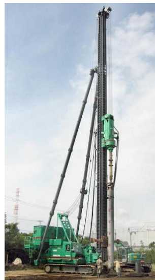
Figure 7.1-4 Three Point Supporting Pile Driver
