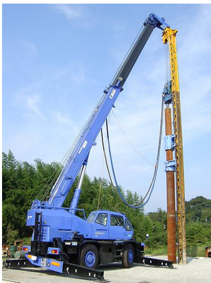
Figure 7.1-3 Suspended Pile Driver
