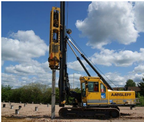
Figure 1.2-4 Pre-cast Pile
