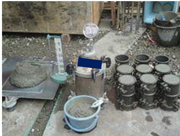
Figure 5.3-22 Testing Concrete on Site
