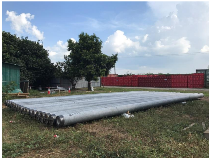
Figure 7.3-14 Storage Condition of Pre-stressed Spun Pile Product
