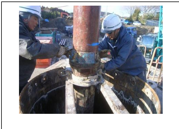
Figure 6.1-25 Flange Type Tremie Pipe
