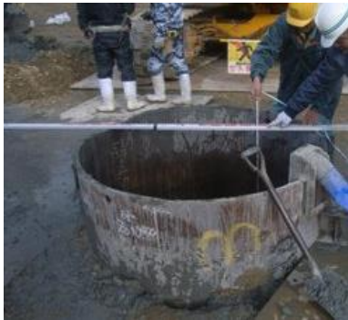
Figure 6.2-21 Measurement of Slurry Sediment
