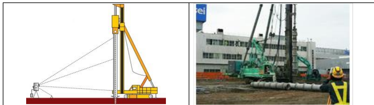
Figure 6.2-13 Drilling Position Survey
