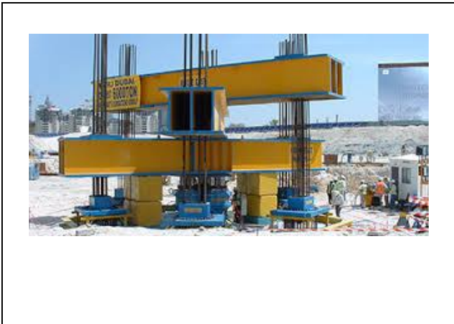
Figure 5.3-13 Static Load Test
