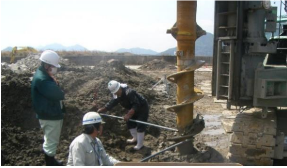
Figure 7.2-7 Measurement of Drill Core Position
