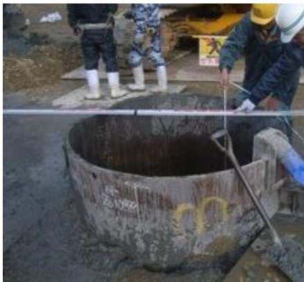
Figure 6.1-12 Confirmation of Excavation Depth
