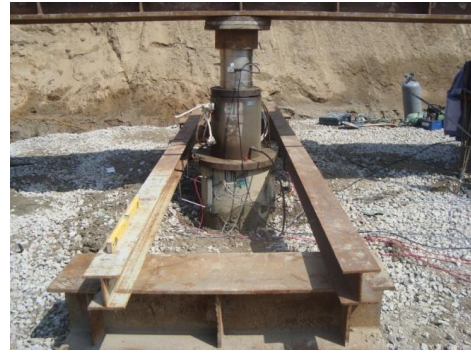
Figure 5.3-2 View of Static Loading Test
