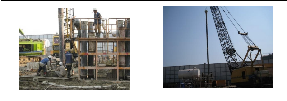
Figure 6.1-28 Tremie Pipe Placement
