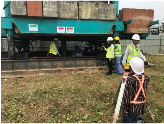
Figure 7.3-23 Measuring for Elevation
