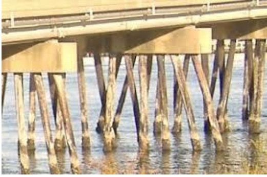
Figure 1.2-2 Timber Pile Foundation
