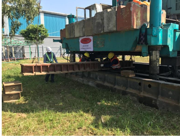
Figure 7.3-31 Preparation of Main Beam onto Machine Body
