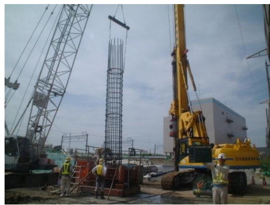
Figure 1.2-5 Cast-in-situ
