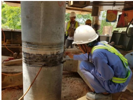
Figure 7.3-27 Welding Work Condition
