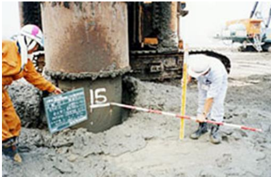
Figure 5.3-23 Measurement of Drill Core Position
