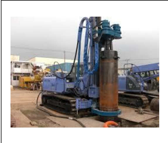
Figure 6.2-11 Settlement of Stand Pipe
