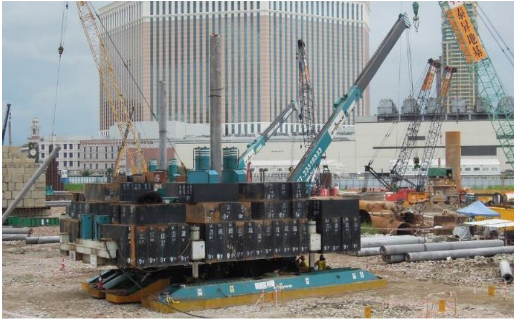
Figure 7.3-15 Pressing Driver
