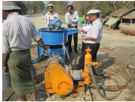
Figure 9.4-1 Example of Mixing Grout in Myanmar
