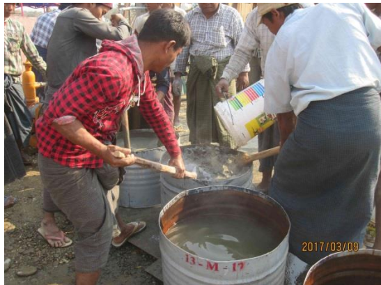
Figure 9.4-1 Example of Mixing Grout in Myanmar
