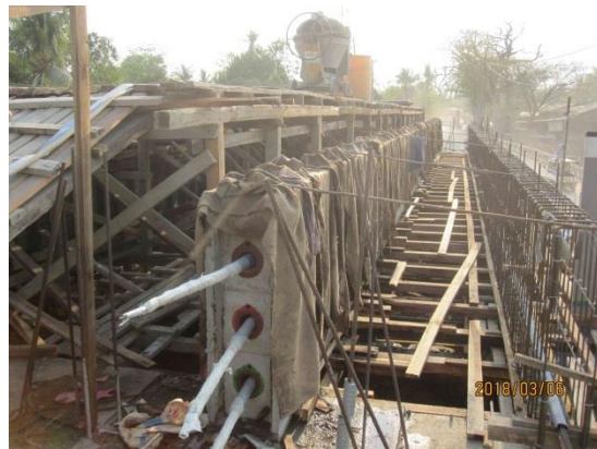
2.1-14 Concrete casting (1): Vibration work for bottom of girder was not enough
