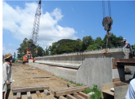
Figure 8.1-2 Prestressing Equipment (Strut Beam) for Post-Tension Girder (At the Site)
