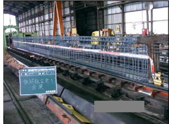
Setting of reinforcing bars
