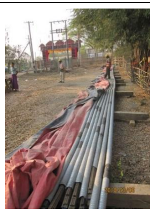
2.1-2 Storage of ducts and PC steel
