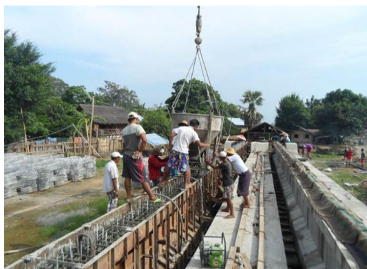
Concreting of Girder
