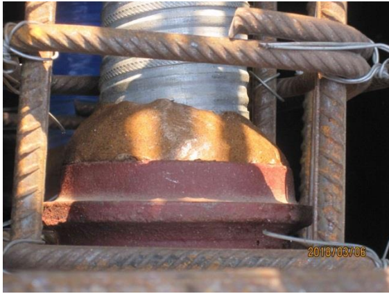
2.1-11 Sealing between duct and anchorage
