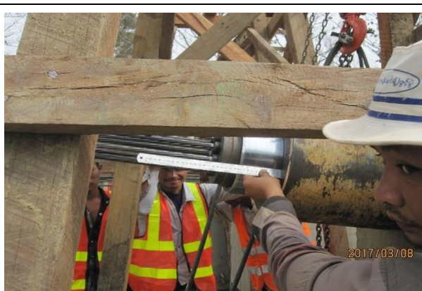
Figure 8.1-7 Measurement of Elongation
