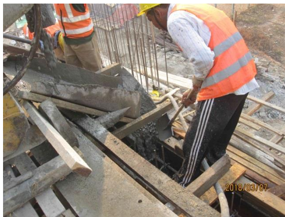
2.1-15 Concrete casting (2)
