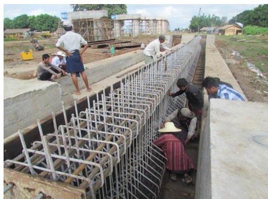
Steel Reinforcement Fixing
