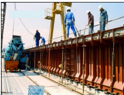
Casting of concrete
