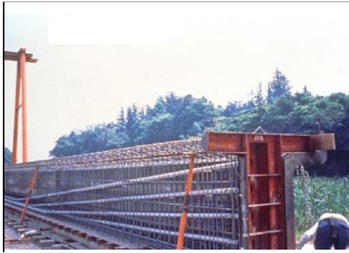
Setting of Re-bars and PC tendon
