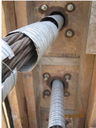
2.1-13 End duct at anchorage (before casting concrete)
