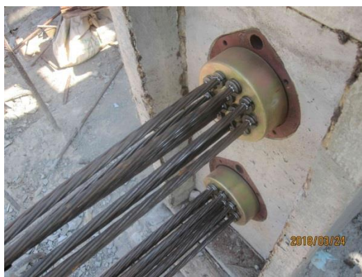
2.2-2 Anchor head before prestressing
