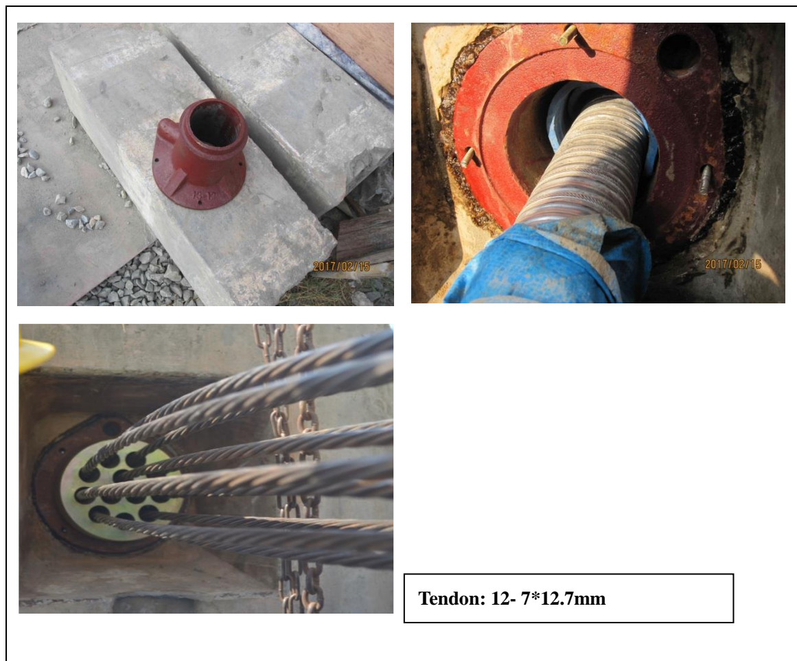
Figure 2.2-2 Typical Anchorage in Myanmar
