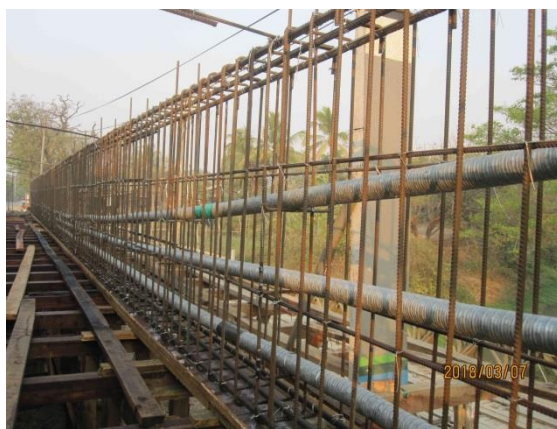
2.1-3 Setting of rebar and ducts
