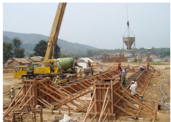
Construction of Strut Beam
