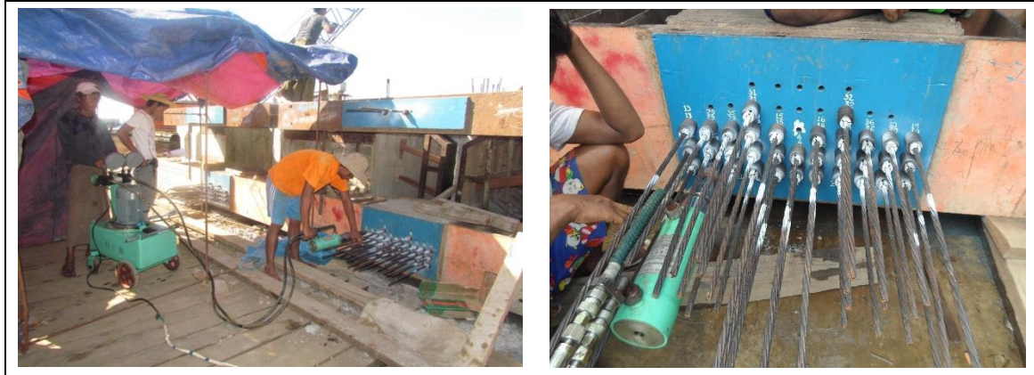
Figure 8.3-1 Tensioning of Pre-tensioning Material (Site Product)
