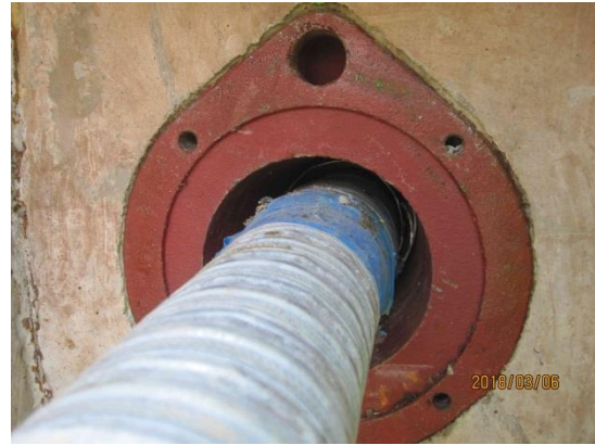
2.1-12 End duct at anchorage (after casting concrete)
