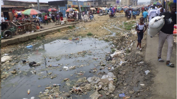
Water ponding with debris in the existing road at around PK4.0 km
