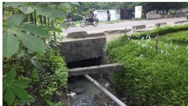
Crossing AG100mm on RHS at PK0.65 km on 16 November 2018
