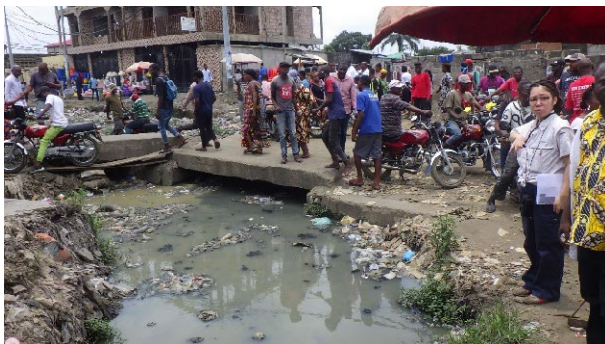
Existing culvert crossing with 3.5m width at around PK3.96 km
