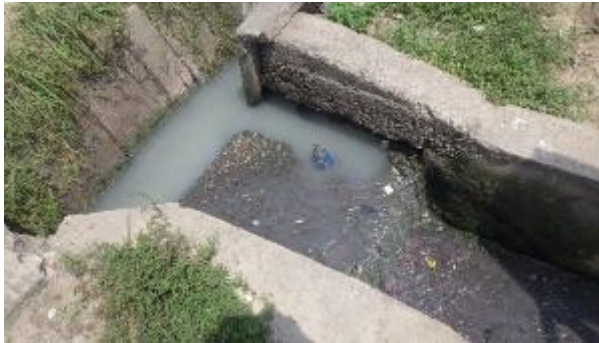
Valve Appeared on RHS at PK0.12 km on 16 November 2018
