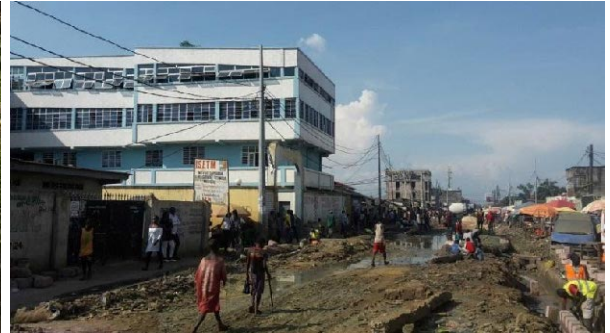
Stagnant water on the road
