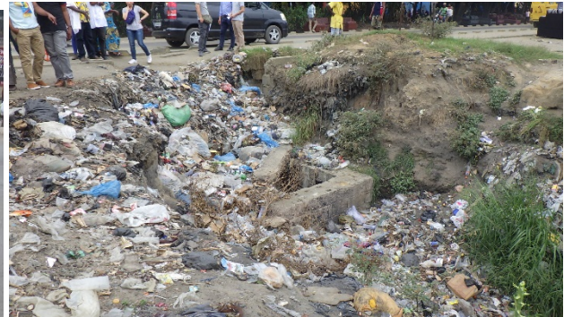
Buried pit and ditch by debris at the drainage crossing at PK2.2 km LHS
