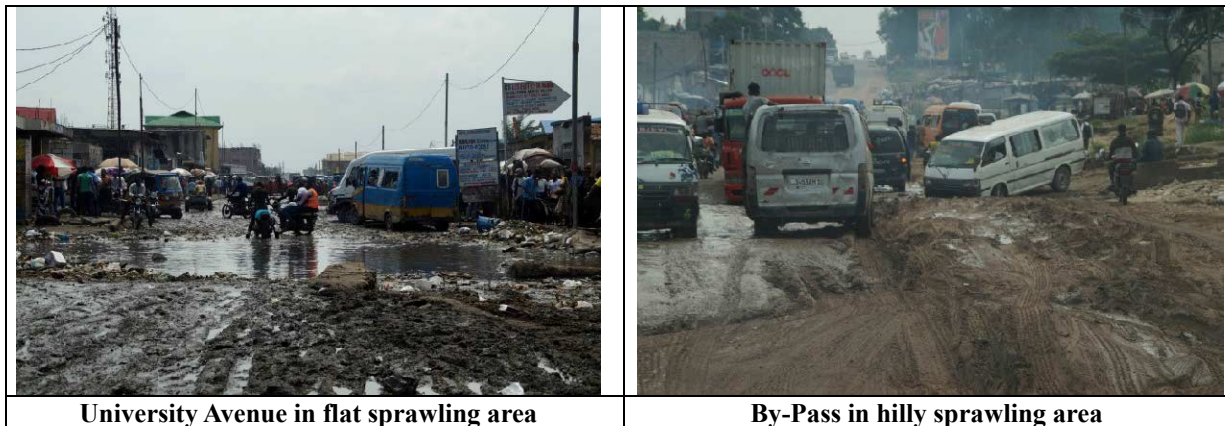
Figure 7.1.9 Current Road Surface Conditions for Target Roads in Study Area
