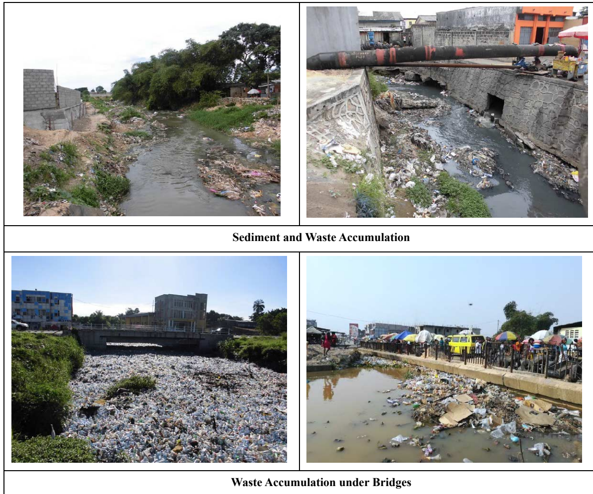
Figure 7.1.12 Reduction of Discharge Capacity
