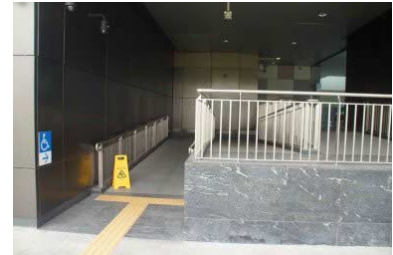
3) Slope facility with handrail at a railway station, Singapore
