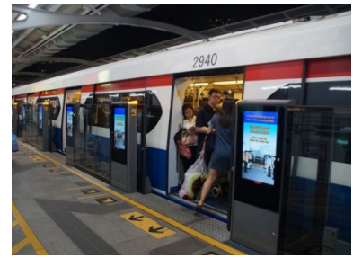
6) Platform door in Bangkok, Thailand
