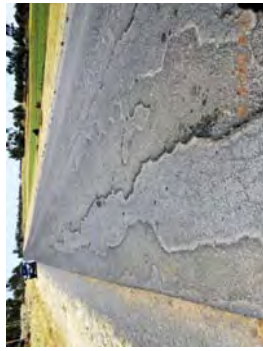
Figure 6.11 Patch Stripping/Exfoliation
