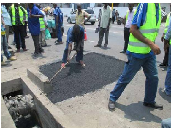
OJT on AP Road Inspection (Patching on Bd. Congo-Japon)
