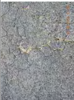
Figure 6.16 Illustration of the Phenomenon of Pumping
