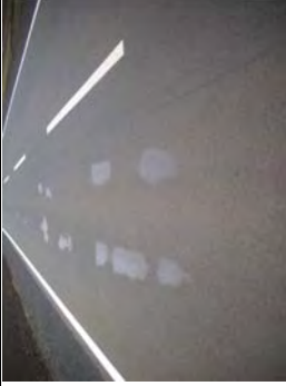
Figure 6.7 Flushing /Bleeding
