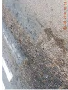
Figure 6.8 Fretting/Raveling
