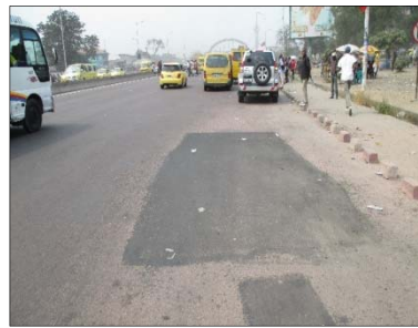
Partial reconstruction of pavement method
