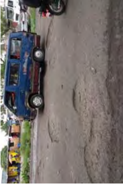
Figure 6.13 Potholes
