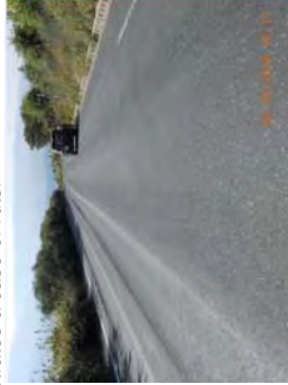
Figure 6.3 Ruts /Rutting
