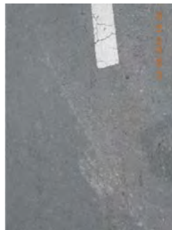
Figure 6.1.a Fine/Hairline Cracks
