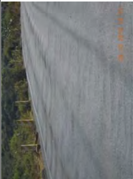
Figure 6.4 Rippling /Corrugation
