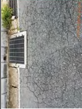
Figure 6.2 Gaps/Faulting
