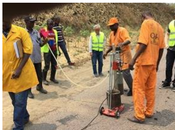
OJT on APm Repair Works RN43 (Sampling)
