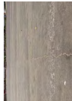
Figure 6.1.b Linear Cracks
