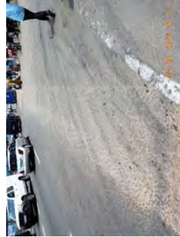
Figure 6.9 Other Example of Fretting/Raveling
