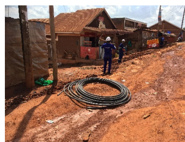
Underground Cable Installation
