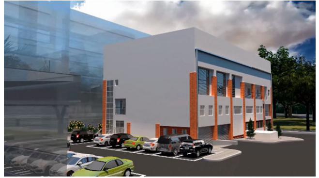
Overview of Traffic Control Centre
