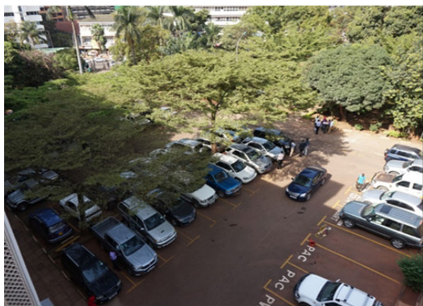
[A] An aerial view of the planned site. It is a flat parking lot (for about 25 vehicles) paved with asphalt. It needs to be demolished and removed for this project.
