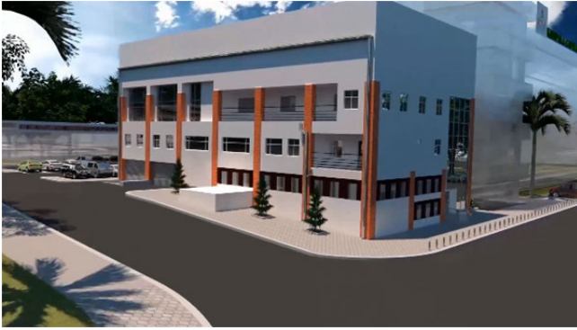
Overview of Traffic Control Centre
