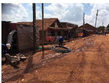
Underground Cable Installation
