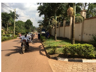
Overhead Cable Installation
