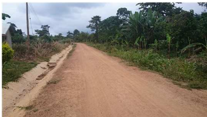
Figure 4-2: Example of Gravel Road in Ghana
