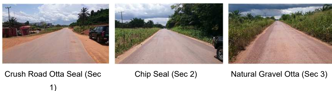
Figure 2-11: The Present Condition of Road Surface at 5 years after implementation
