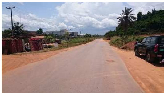
写真-1 Crush Road Otta Seal (Sec 1)
