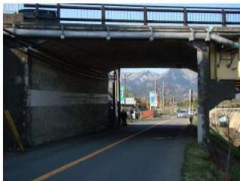
Rigid-Frame Abutment
