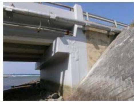
Inverted T-type Abutment
