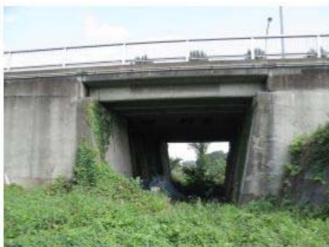
Gravity Type Abutment
