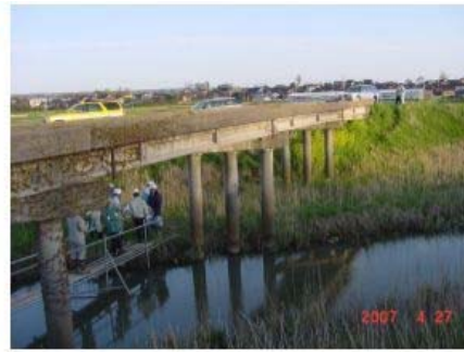
Pile Bent Bridge Pier
