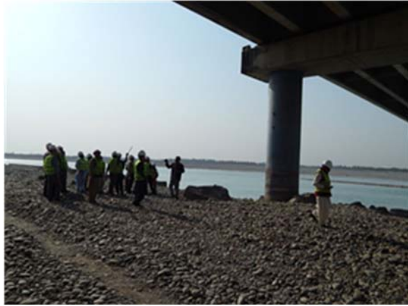
Indus River Bridge
