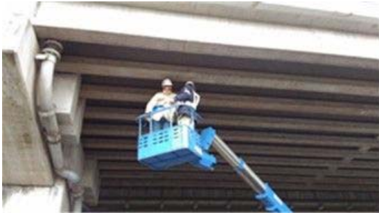
Ride on Bridge Inspection Car
