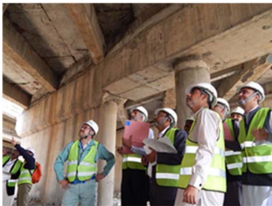
Wah Garden Bridge
