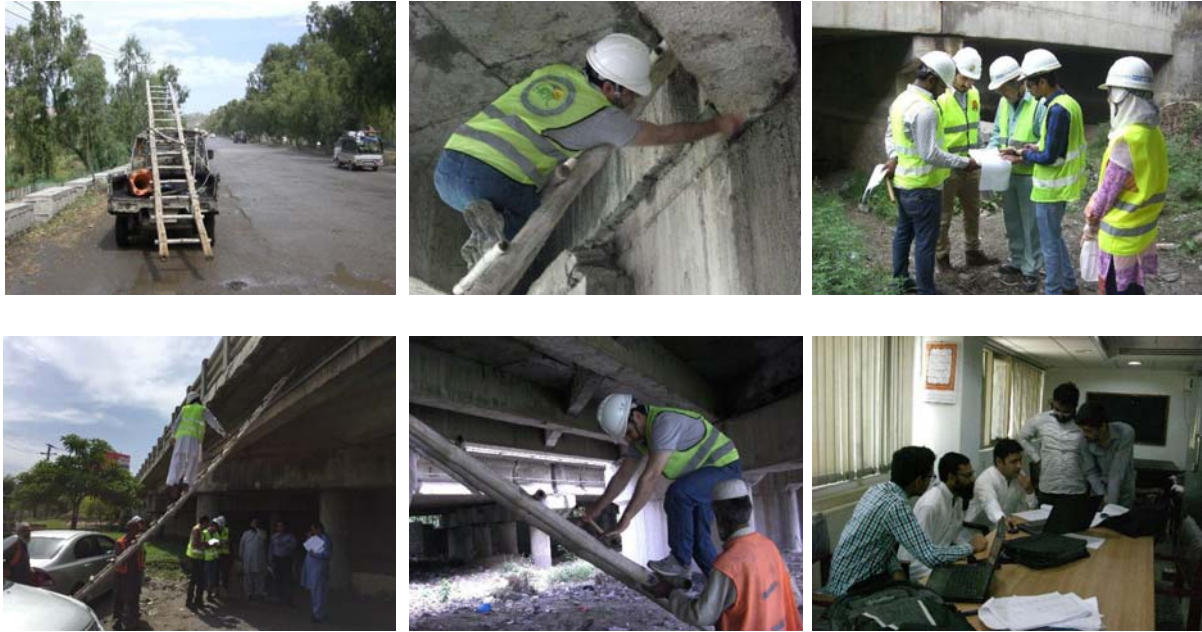
Figures: Accompanying and guidance to the site work
