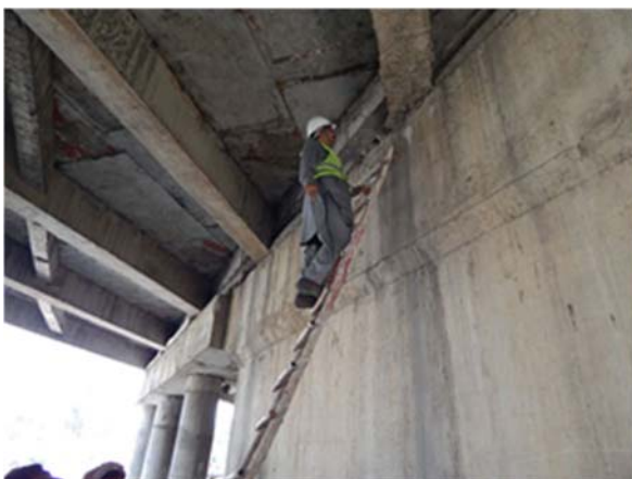
Wah Garden Bridge
