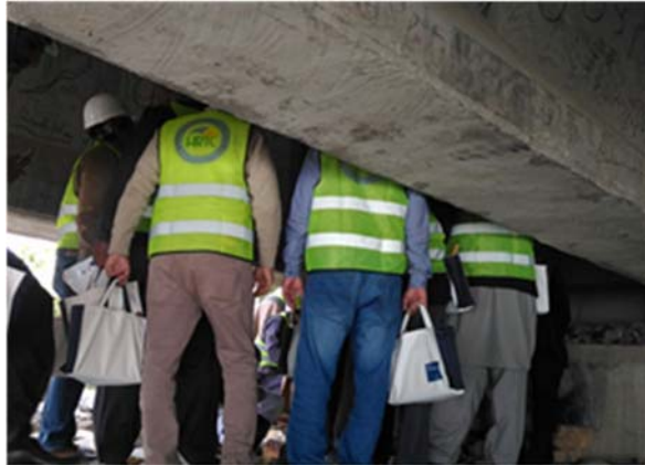
Indus River Bridge
