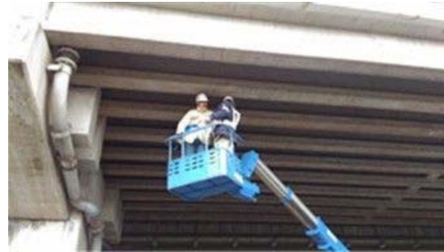
Lift car for bridge inspection
