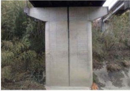
Hammerhead Pier
