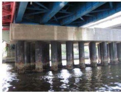
Pile Bent Bridge Pier
