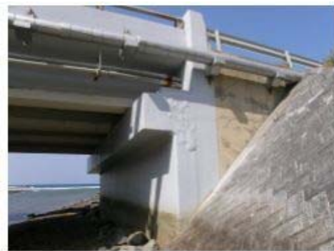
Invented T-type Abutment
