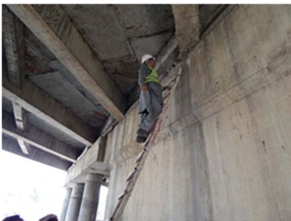
Wah Garden Bridge
