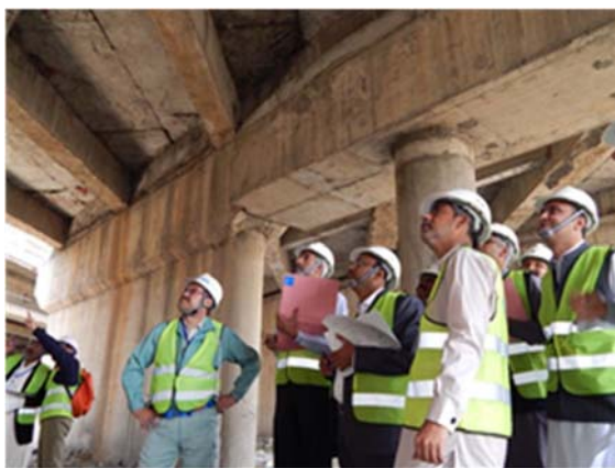
Wah Garden Bridge
