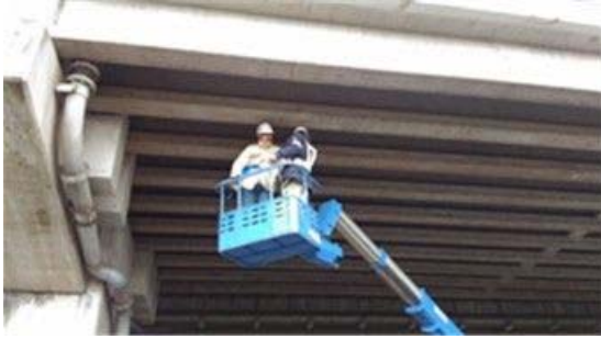
Ride on Bridge Inspection Car
