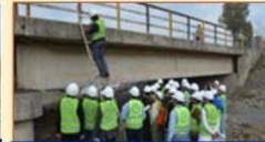
Site Visit (Shahia Bridge)
