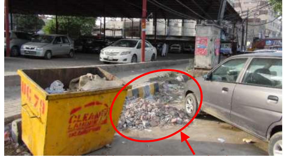
PTCL installed cable and did not put back to its original form
