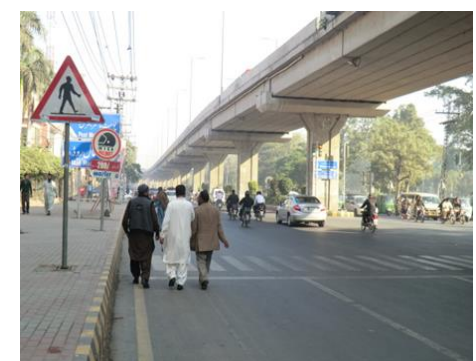
④ Pedestrians walking on the carriageway under the N5 overpass
