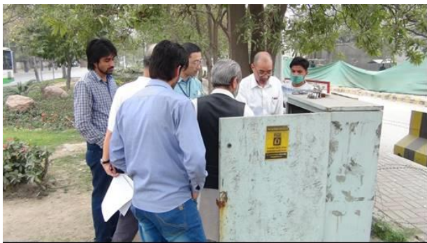
On-site training of signal controller
