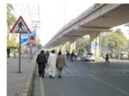
④ Pedestrians walking on the carriageway under the NS overpass
